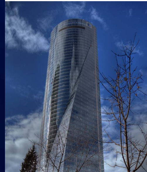
Torre Espacio Building, Madrid, is automated using self-powered wireless network of 4200 switches, 13500 addressable luminaries and 4500 blinds
